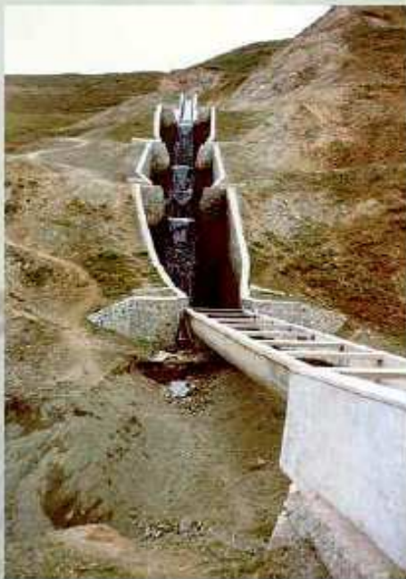
Conveyance canal in Qinghai Province, China
